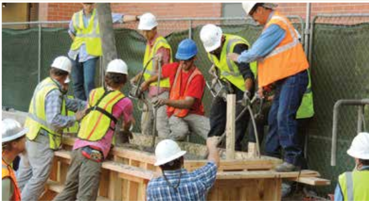
During the first large concrete pour, UAFM staff worked alongside the students, teaching them proper technique for placing and finishing concrete. During the second pour, students performed most of the labor with supervision by UAFM staff. During the third pour, the students worked with minimal supervision by UAFM staff. (Photo by Mark Marikos)
